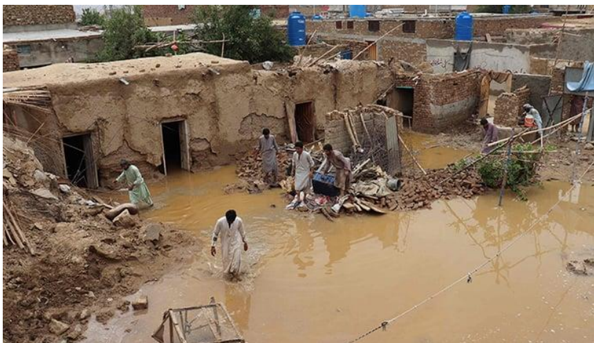
Figure 4: Residents clear debris of damaged houses after heavy monsoon rainfall.
