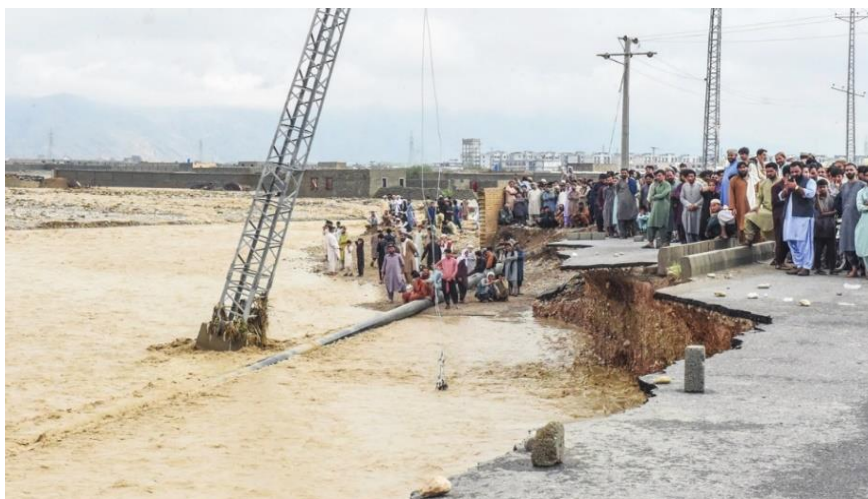
Figure 5: Bypass Road towards Hanna Lake after the flash floods
